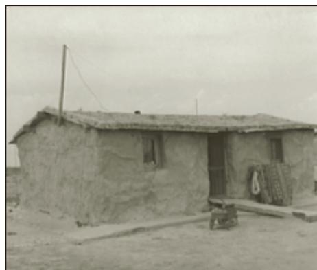
Sod houses like this were home to farmers on the Nebraska prairie.
