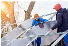
install a system
